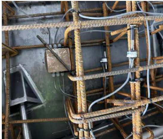
Figure 2-1 VibraLink Hex installed in tunnel segment monitoring array
